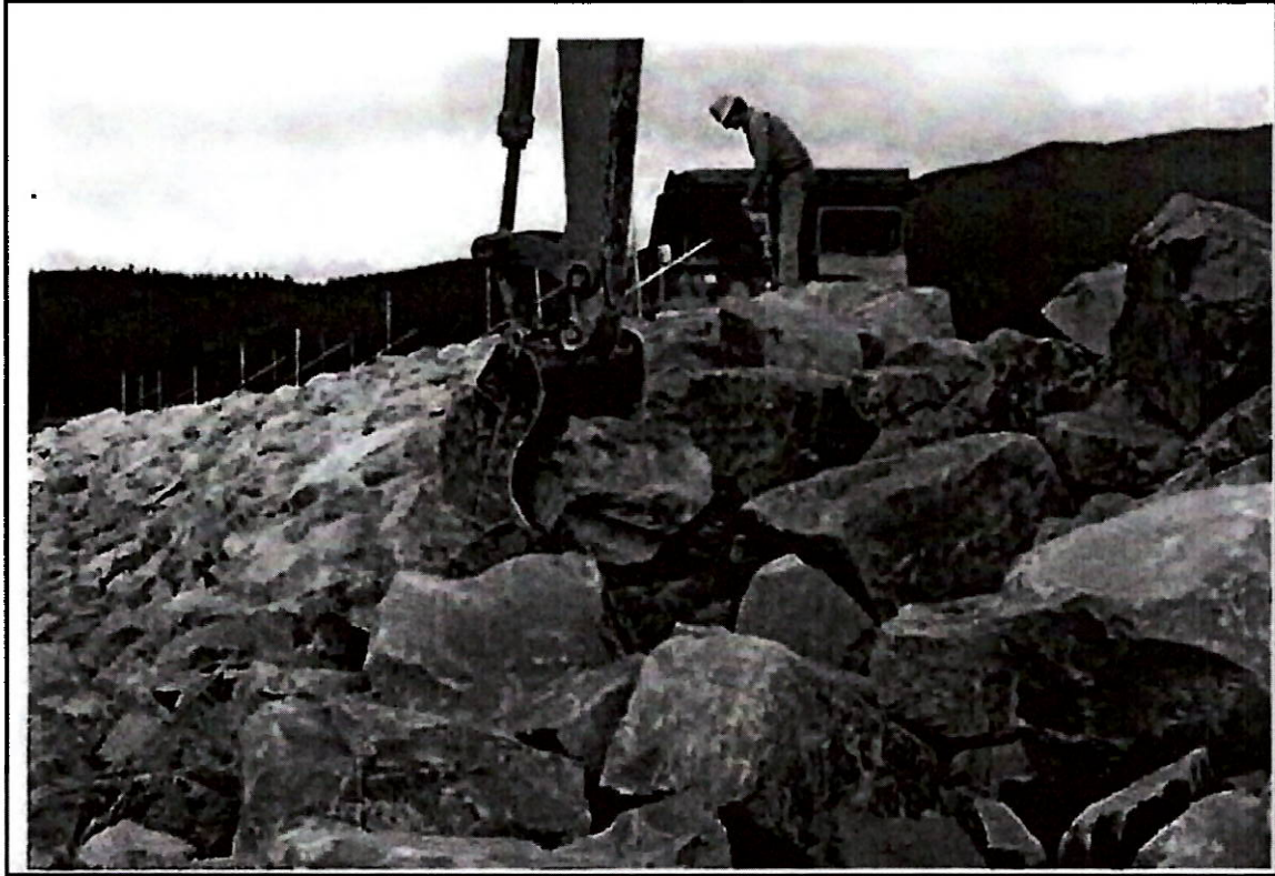
Figure-30: Placement of Riprap as slope stability on the upstream side.
