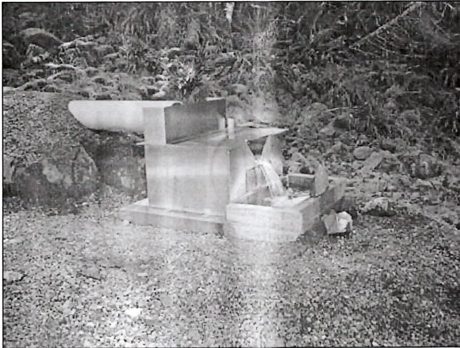
Dam Seepage Measuring Stainless Steel Weir Box
